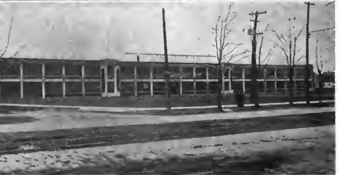
Three examples of modern automobile factory construction to be seen in Detroit. The buildings, besides being large and spread out over a considerable area, are designed to afford plenty of light and air for the workmen
